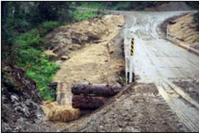
Figure 3. Hay mulch and seeding used for erosion control at a stream crossing.
