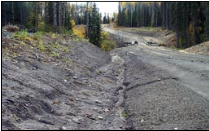
Figure 1. Sediment generated from a long ditch line that flows directly into a stream at a road crossing (this photo is not from the Lamprey Creek watershed).
