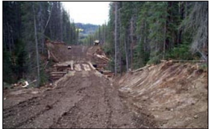
Figure 5. New bridge crossing – site PC030.
